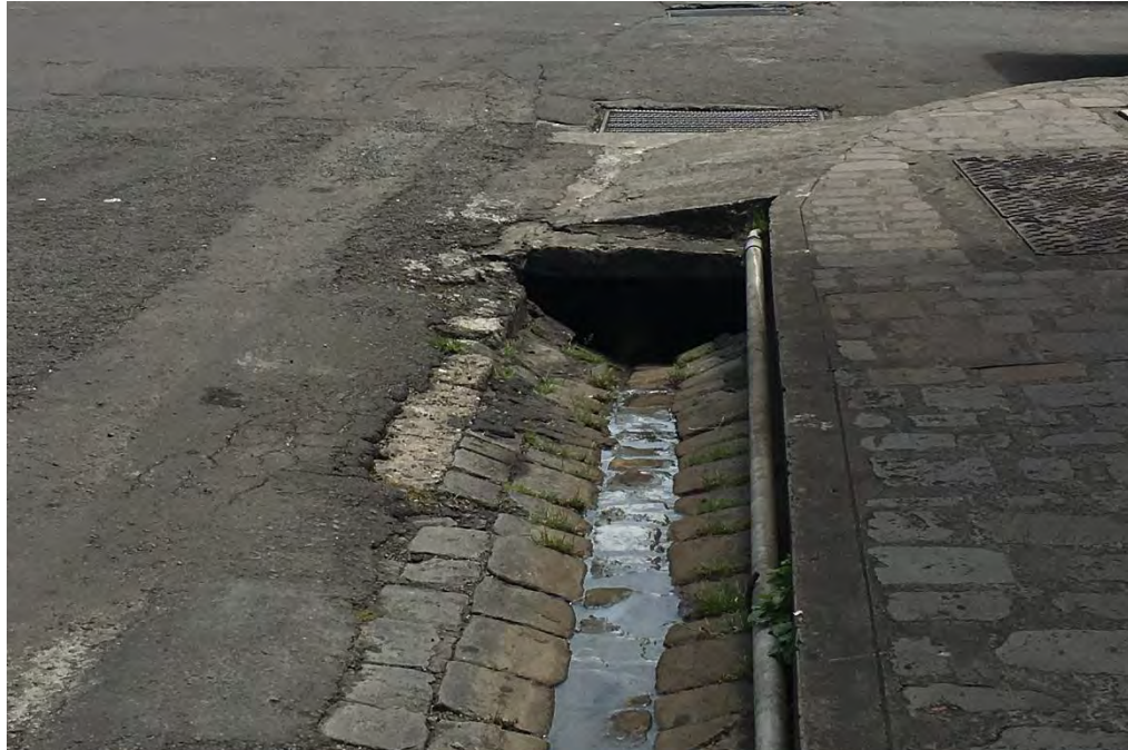
Figure 4: Example of Stormwater Conveyance in the Kingstown Port Area
