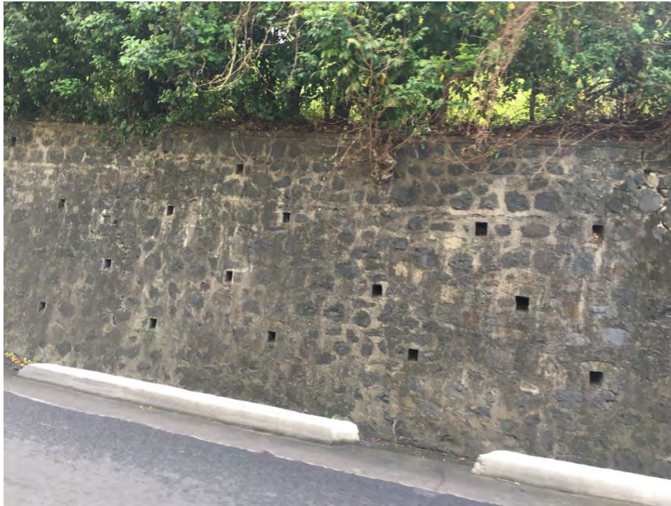
Figure 5: Example of Stormwater Conveyance in the Kingstown Port Area
