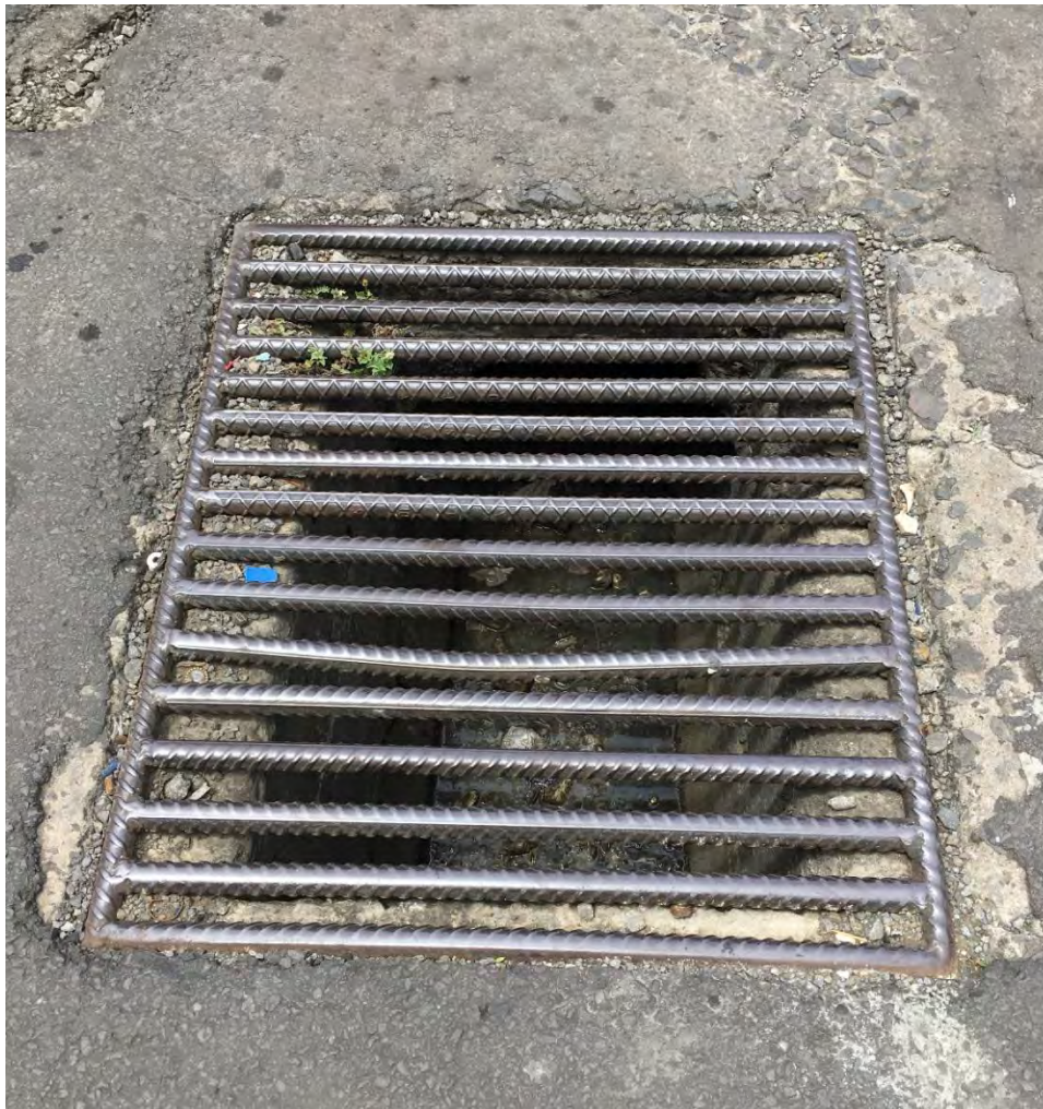
Figure 6: Example of Stormwater Conveyance in the Kingstown Port Area
