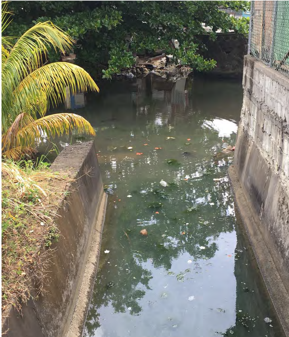
Figure 7: Example of Stormwater Conveyance in the Kingstown Port Area
